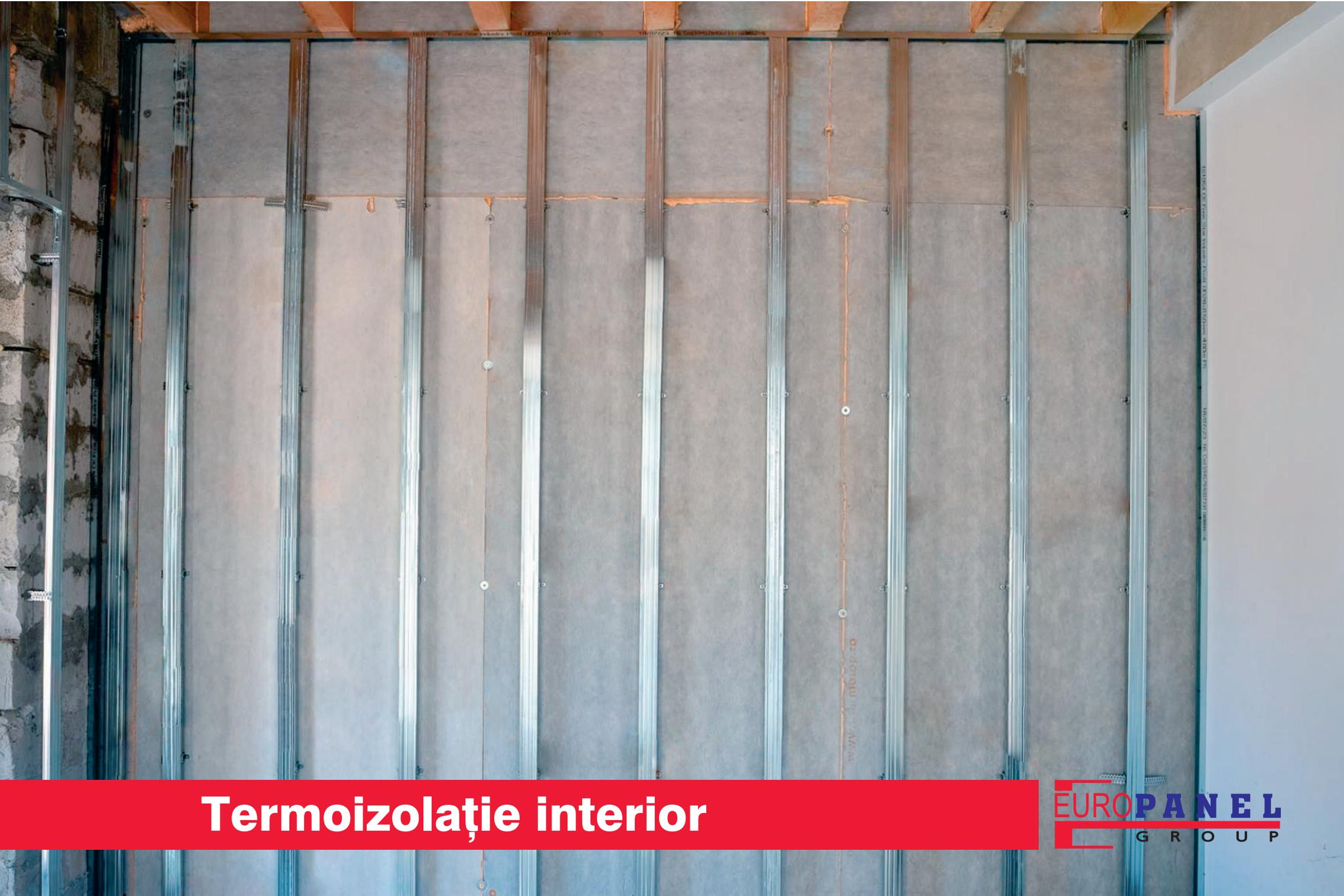
The image shows a cross-section of an interior wall during the insulation process. A metal frame of vertical studs is visible, with a grey mineral wool insulation material being installed between them. The studs are secured with screws. On the left, a portion of the existing brick wall is visible. At the bottom, there is a red banner with white text. In the bottom right corner, there is a logo for 'EUROPANEL GROUP'.
